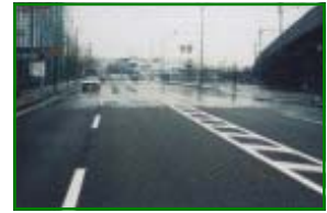
Front: Modified-asphalt high-drainage paving. Rear: Conventional asphalt paving.
