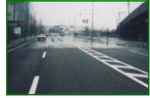
Front: Modified-asphalt high-drainage paving. Rear: Conventional asphalt paving.
